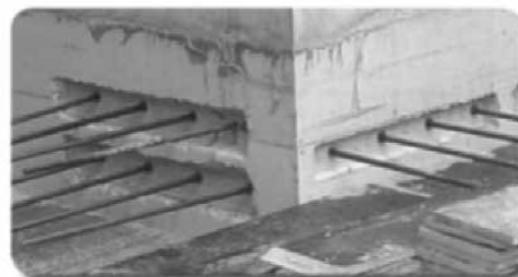
ReidBar™ Inserts installed in the ReidBox rebate former
