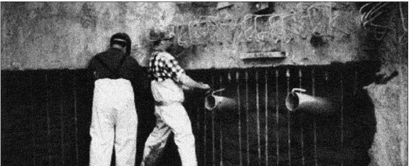
Retaining walls constructed from the top down.
