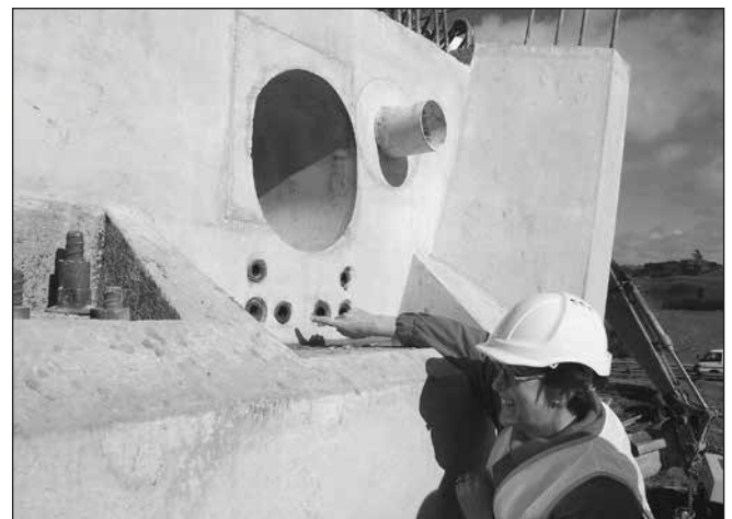
Structural connections using RB32 couplers in bridge construction.
