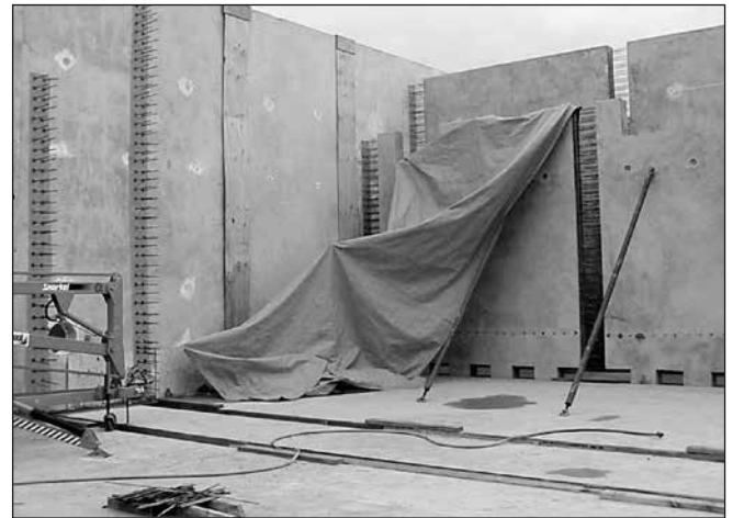
RB12 threaded inserts anchoring starter bars at a new water treatment facility.
